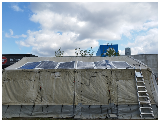
MSF is developing a solar energy rapid deployment kit that can be installed on the roof of tents commonly used in emergency responses, with the capacity to supply 9 kWh/day of electricity.
